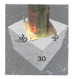
With plint: an excavation dig with the right dimensions for the main poles is necessary. Make a glush of concrete in the dig before fixing the plates with dowels.
